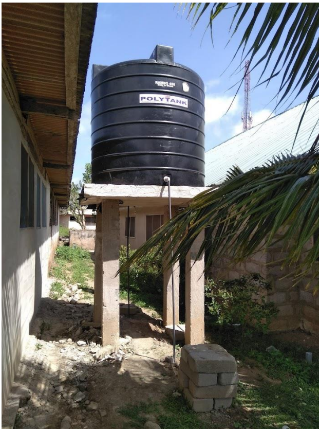
Picture 15: Polytank for for storing water at sachet water production site, Cape Coast
