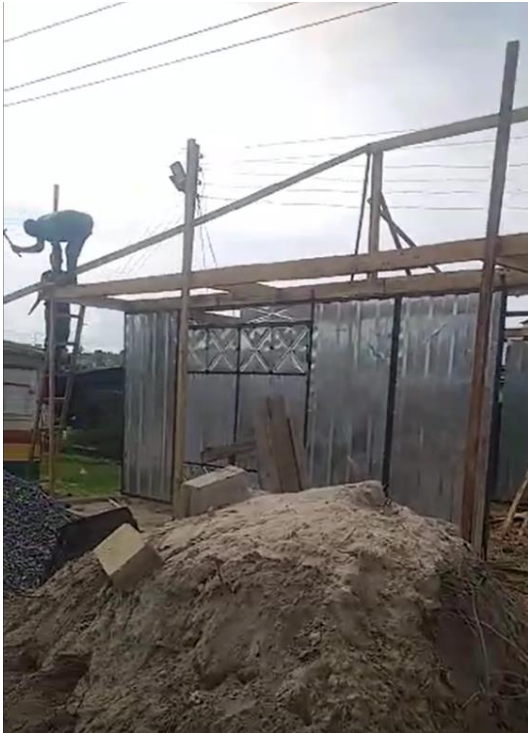
Picture 1: Roofing of the milling centre at Amponsah Market, Suhum
