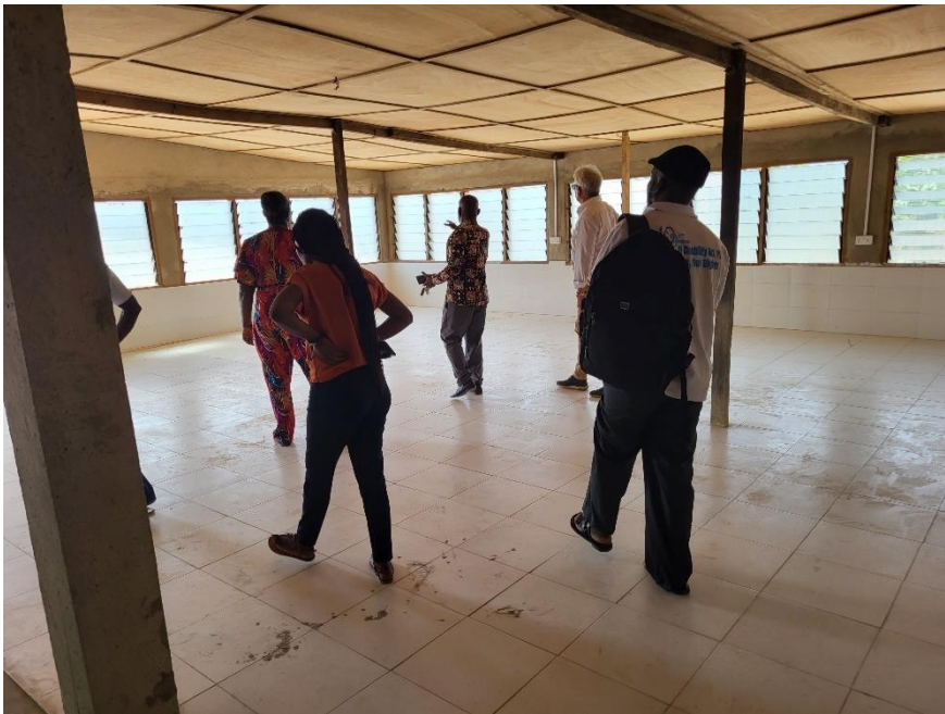
Picture 13: Sachet water production site after reconstruction, Cape Coast
